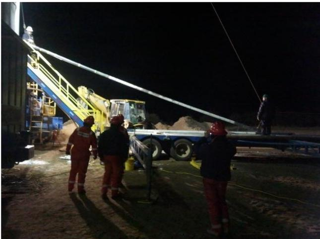
**Figure 4: The whole BHA being lifted into position showing overall length**
